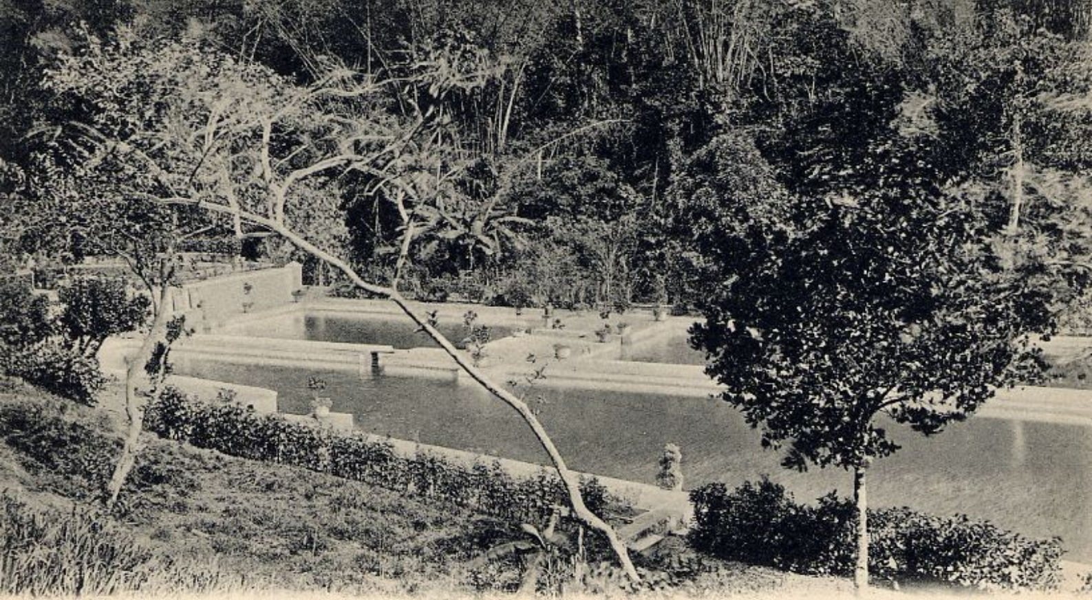
Maraval Reservoir, Trinidad, B. W. I.
