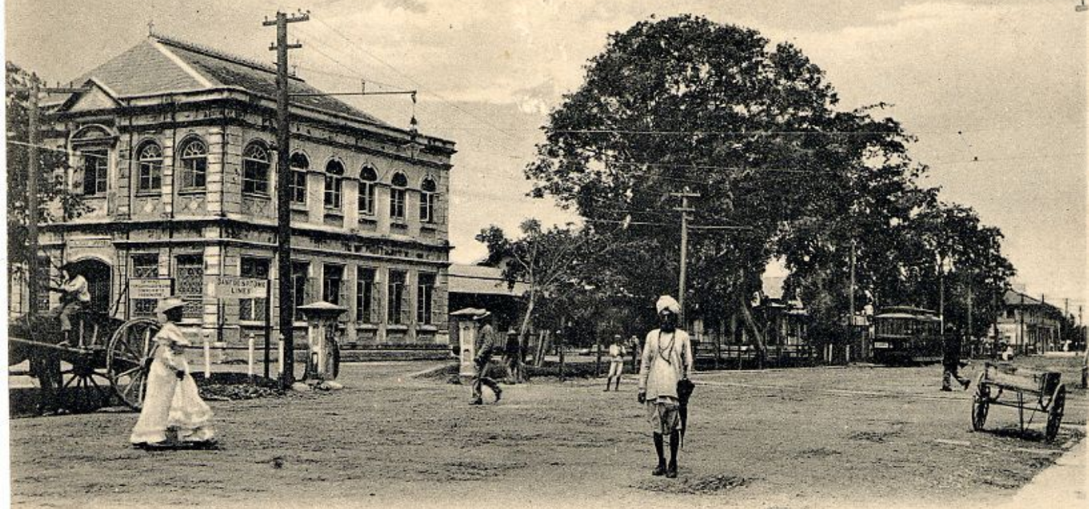
Railway Offices. Trinidad. B. W. I.
