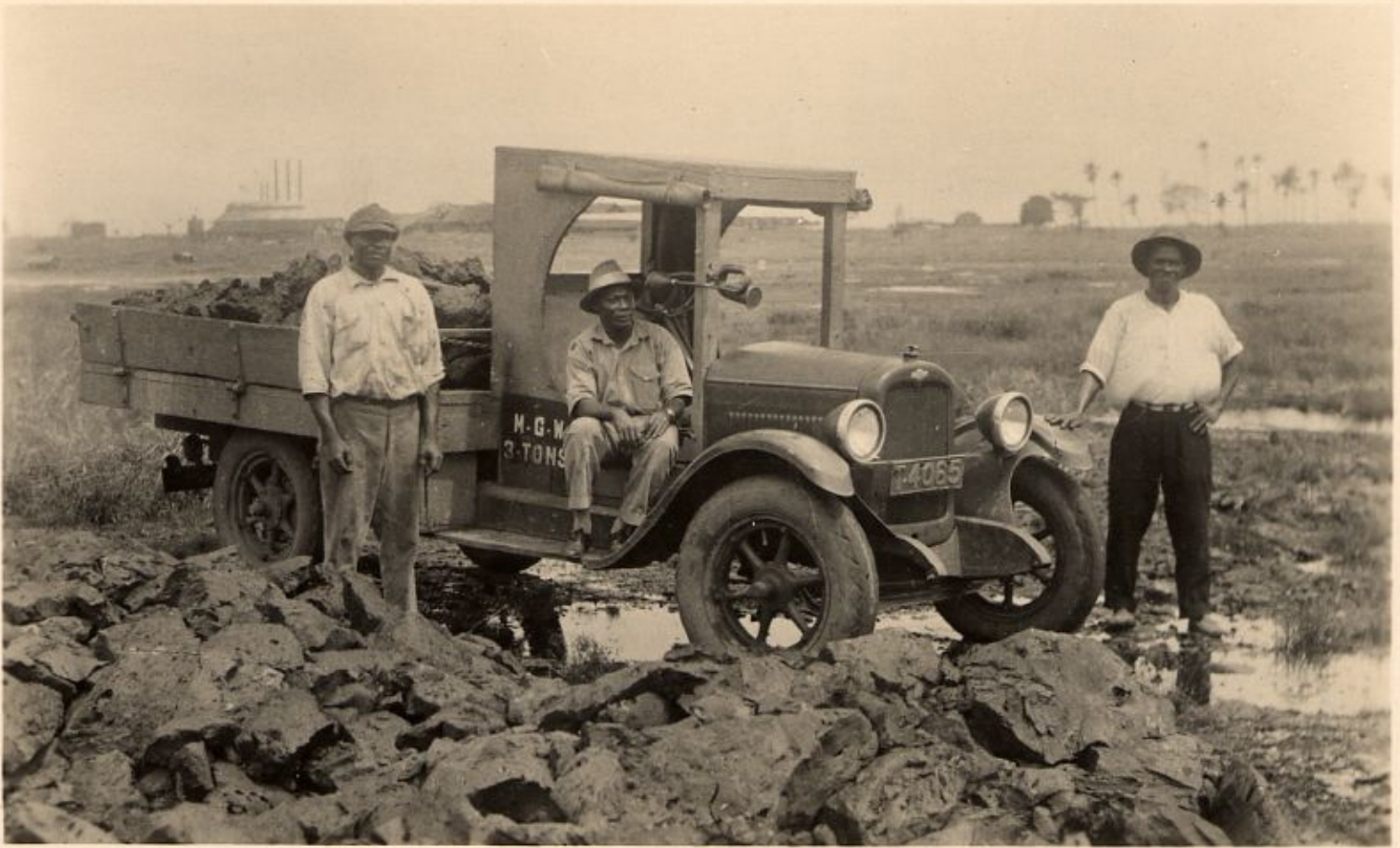
LOADING PITCH, LA BREA, TRINIDAD, B.W.I
