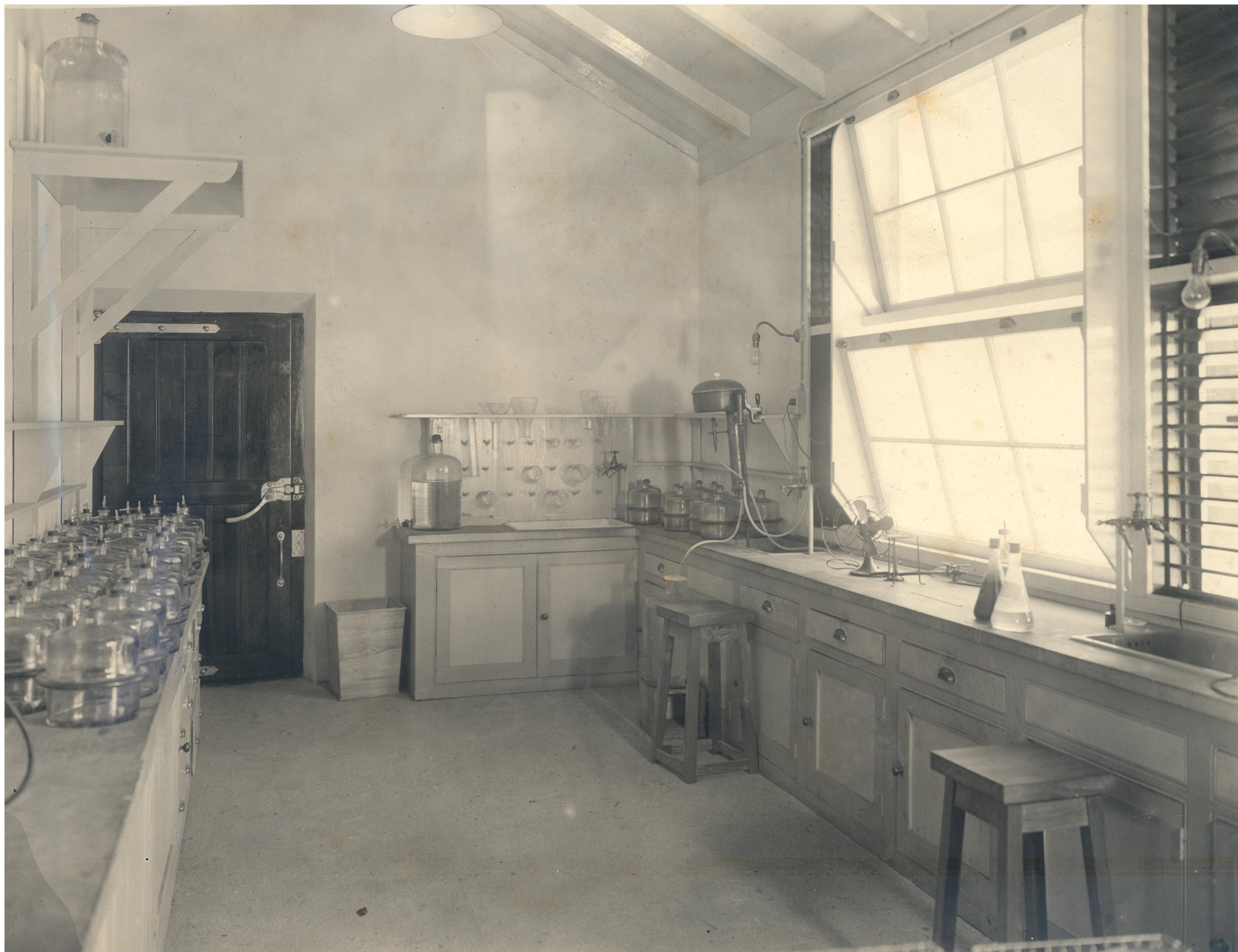
North end view of Lower Temperature Laboratory
