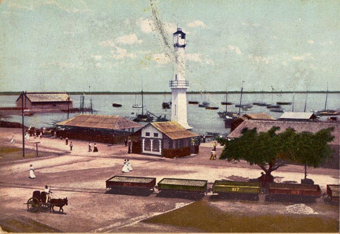
Light House and Produce Sheds Port of Spain Trinidad.
