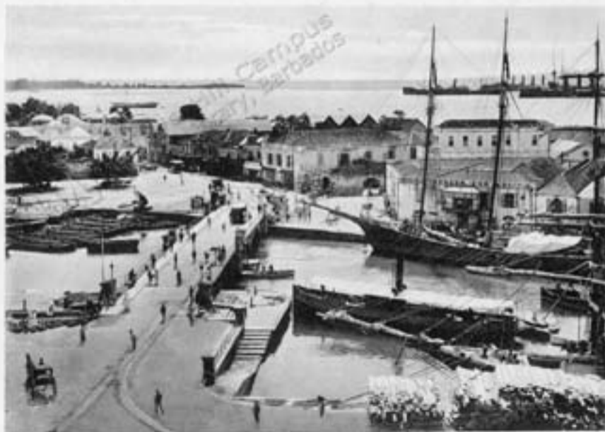
Bridgetown, Barbados. Showing Swing Bridge and outer harbour.
