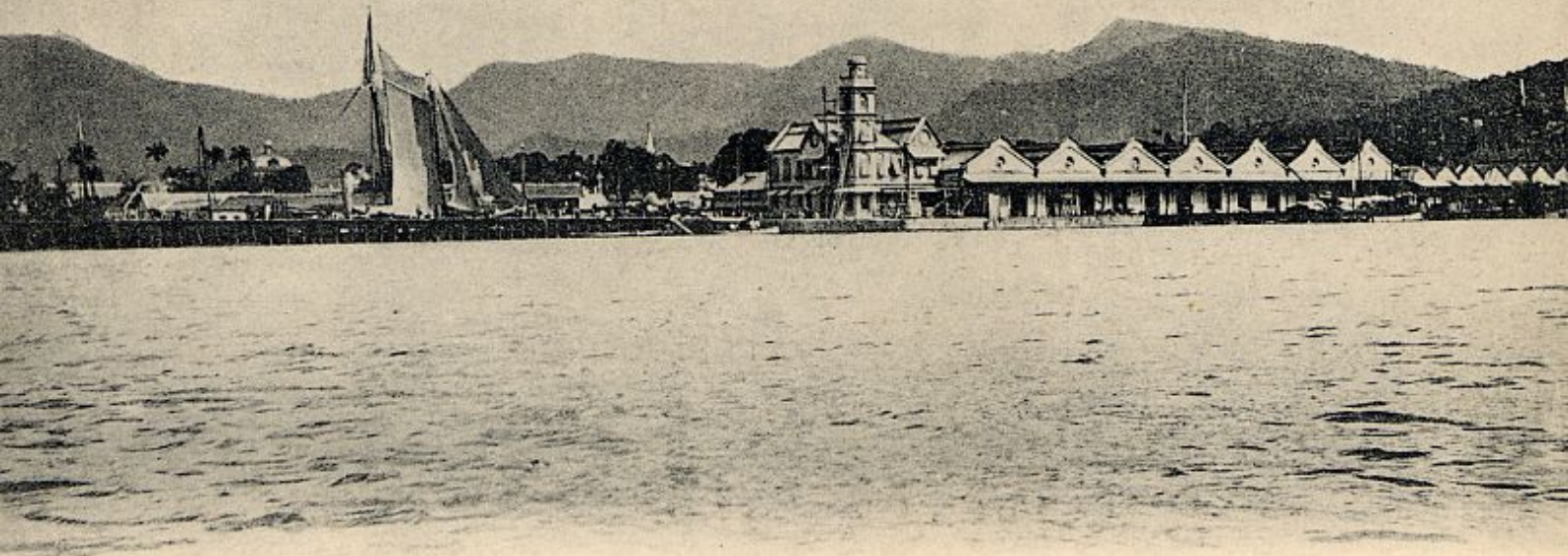
Customs and Landing Wharf, Trinidad, B.W.I.
