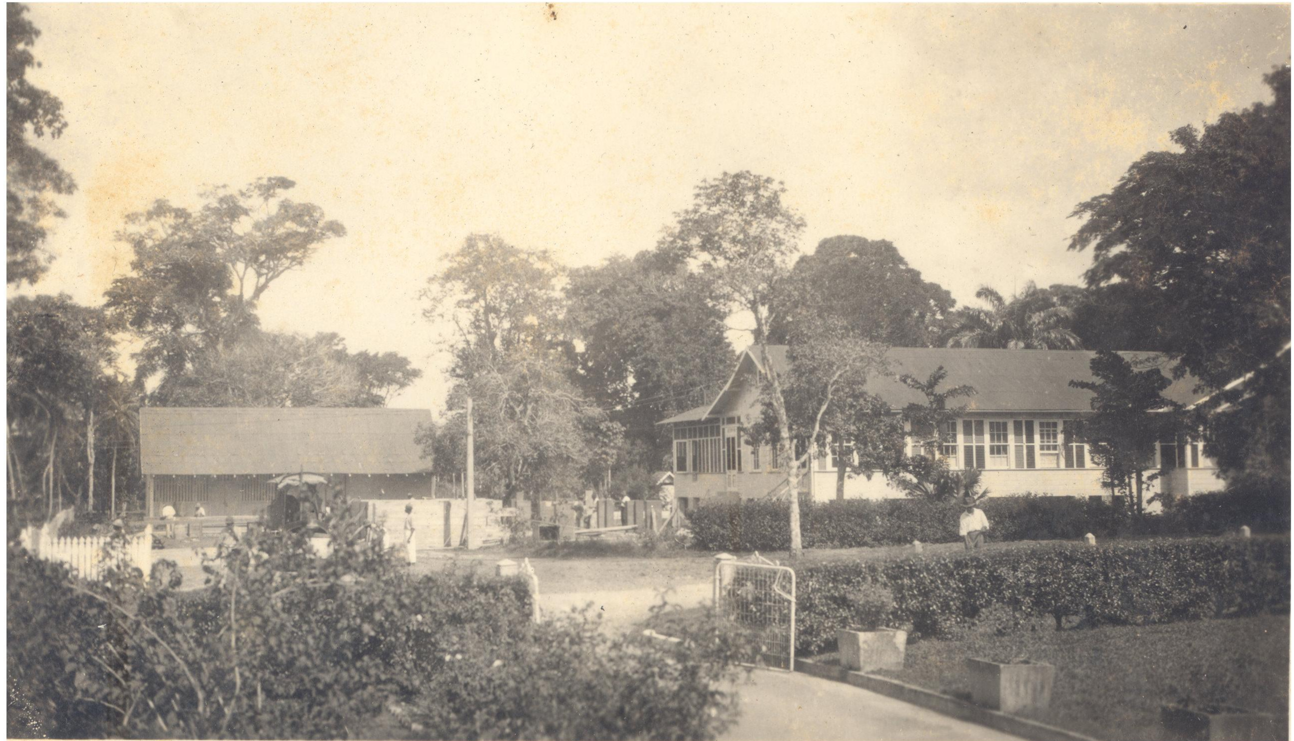
Gallery extension to Drawing Room of Principals' House — December, 1925
