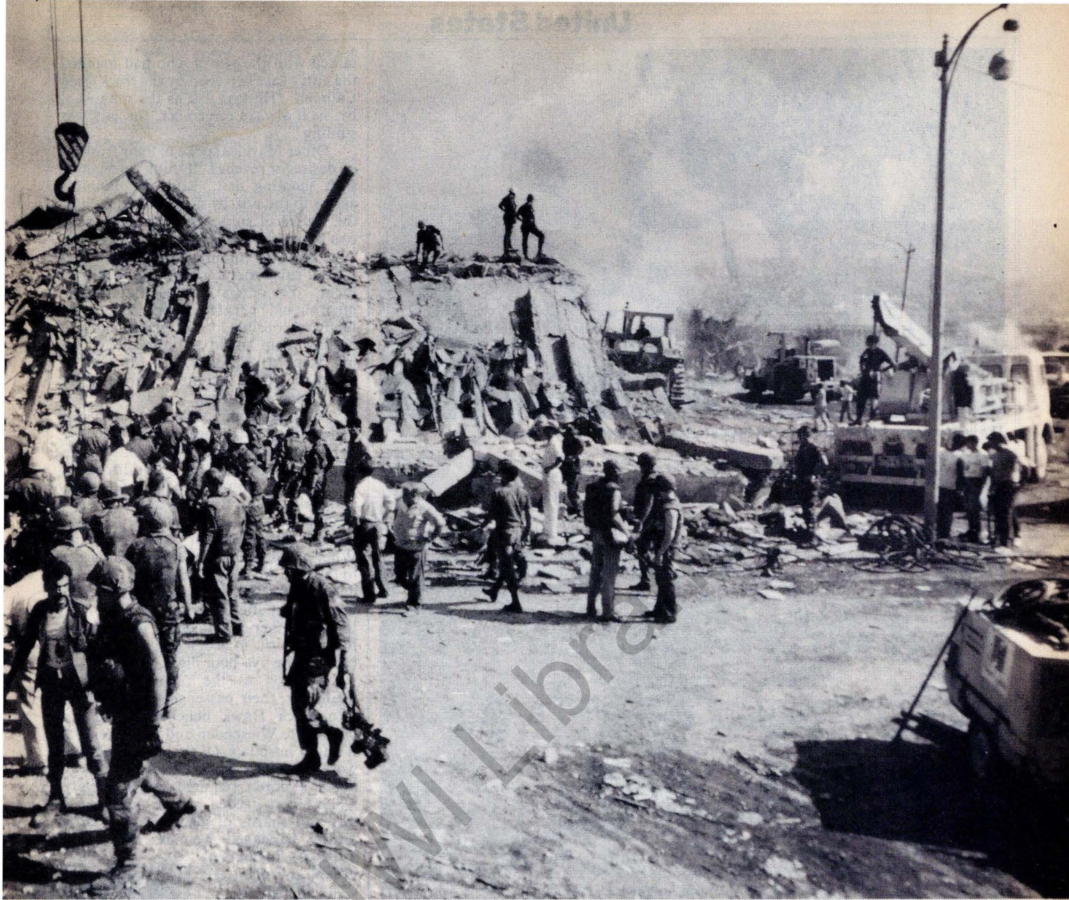
workers, gingerly pull apart the grotesque tangle of concrete and steel as they search for fallen comrades
