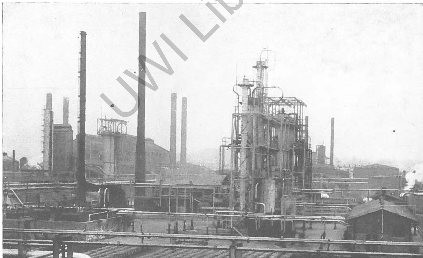
ESTER SALTS PLANT — STANLOW REFINERY
