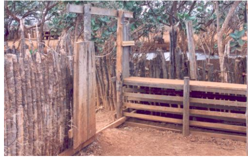
Figure 92: Swing gate at side of the wooden chute
