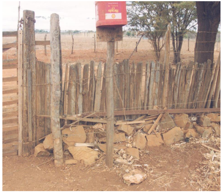
Figure 67: Fencing arrangements showing the red plastic box protecting the electric fencing impulse generator.
