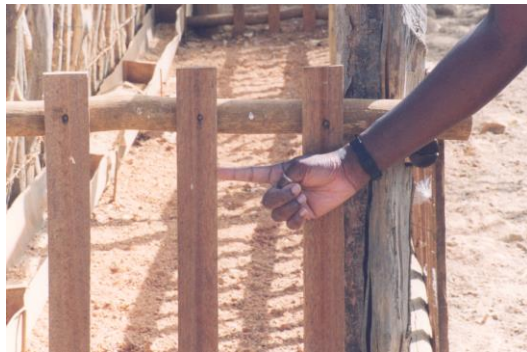
Figure 76: The spacing between the verticals in the creep feeding area is about 12 cm
