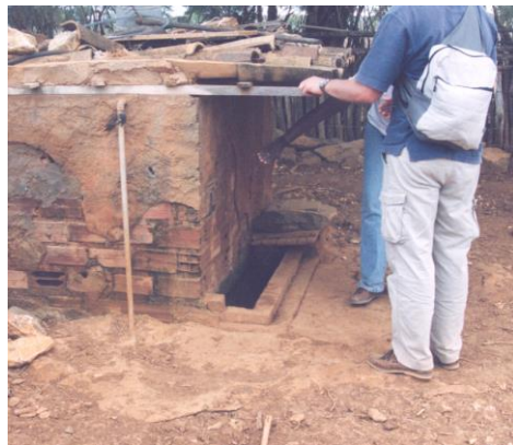
Figure 71: Older brick water tank and drinking trough that is about 15 cms wide, the young sometimes fall into this trough.
