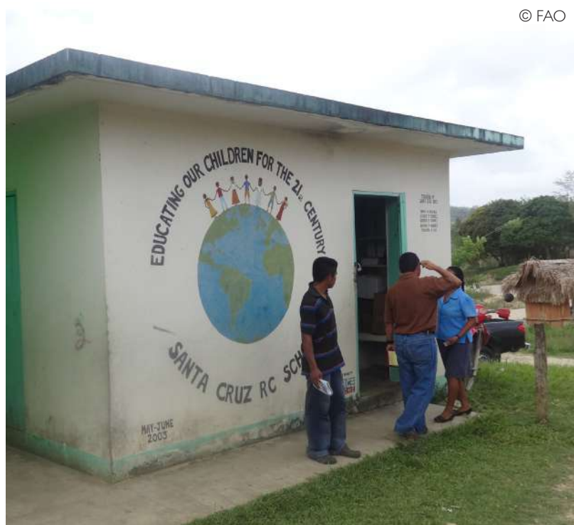
Old kitchen and storage room, July 2016.
