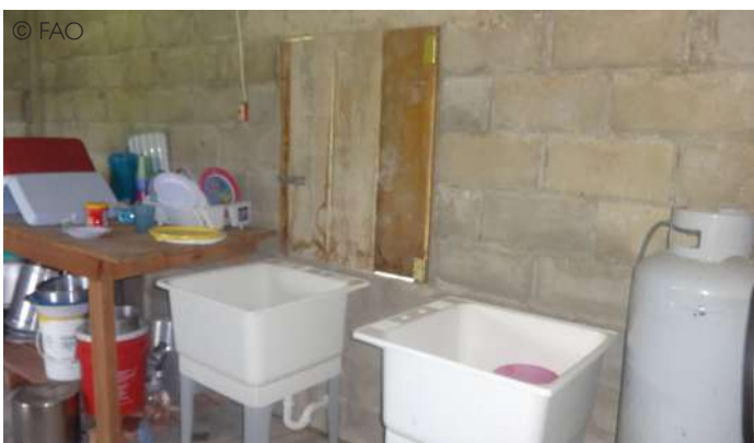
Old kitchen area, July 2016.
