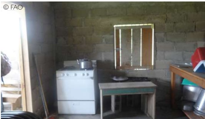
Old kitchen area, July 2016.
