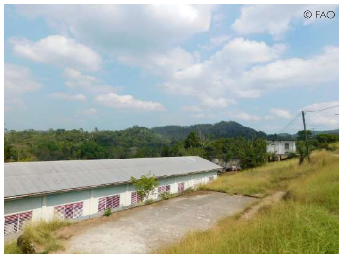
New kitchen, storage and lunchroom infrastructure, November 2017.
