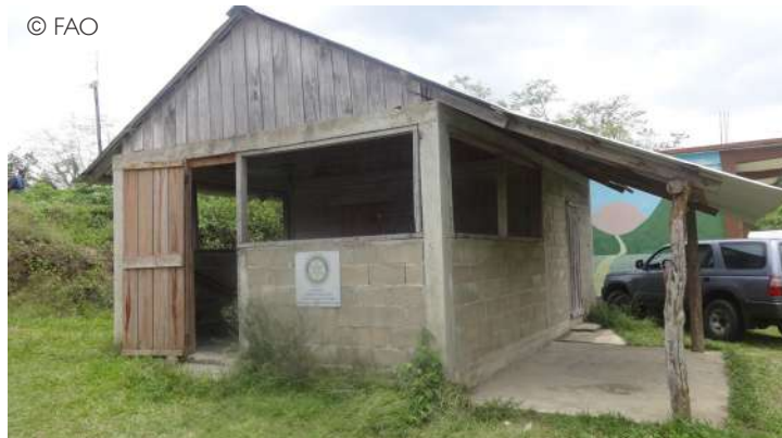
Old kitchen infrastructure, July 2016.
