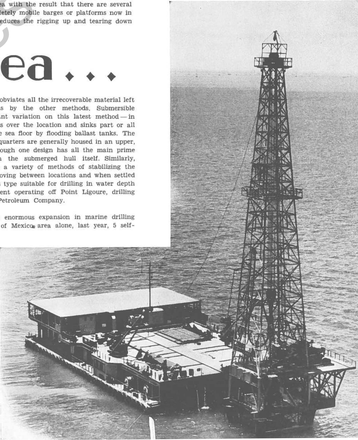
Right : Typical small permanent platform and drilling tender.
