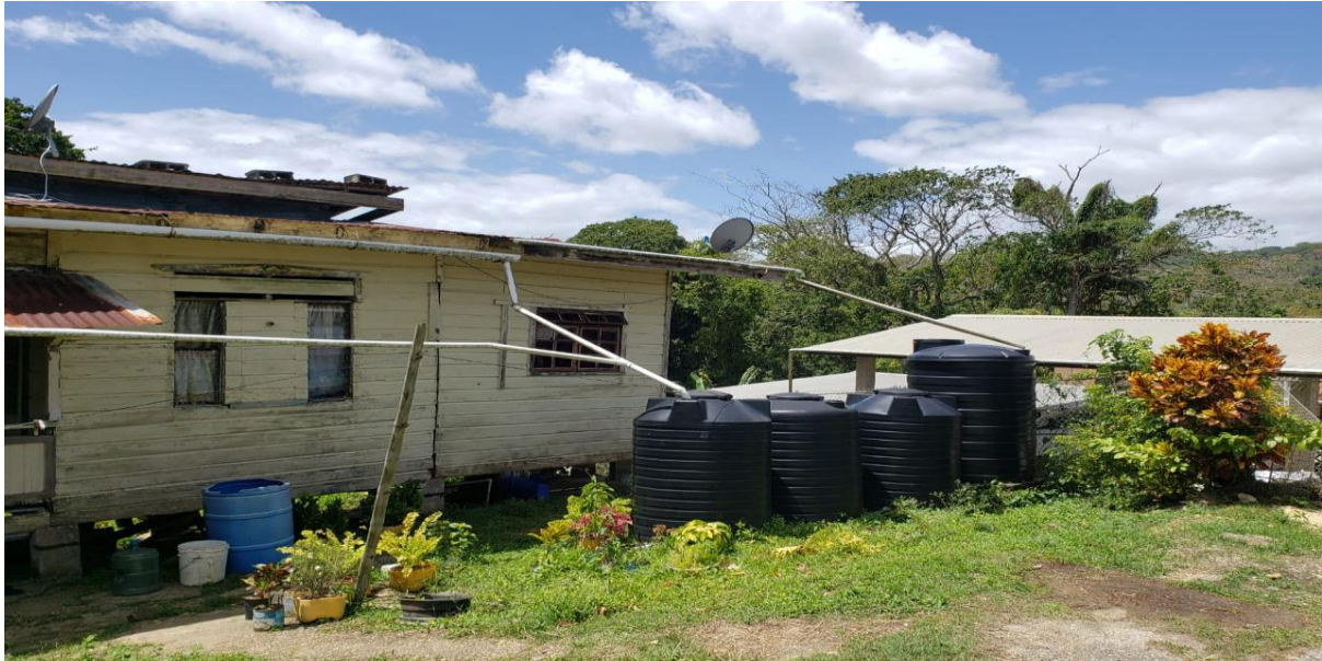
Figure 9 - Tanks being used by a household in Corosal in harvesting rainwater
