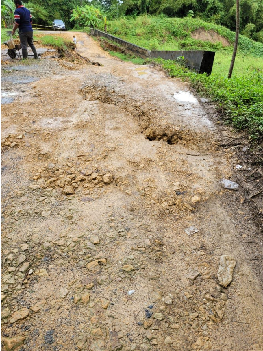
Figure 13 - Community self-help spirit in repairing poor roads
