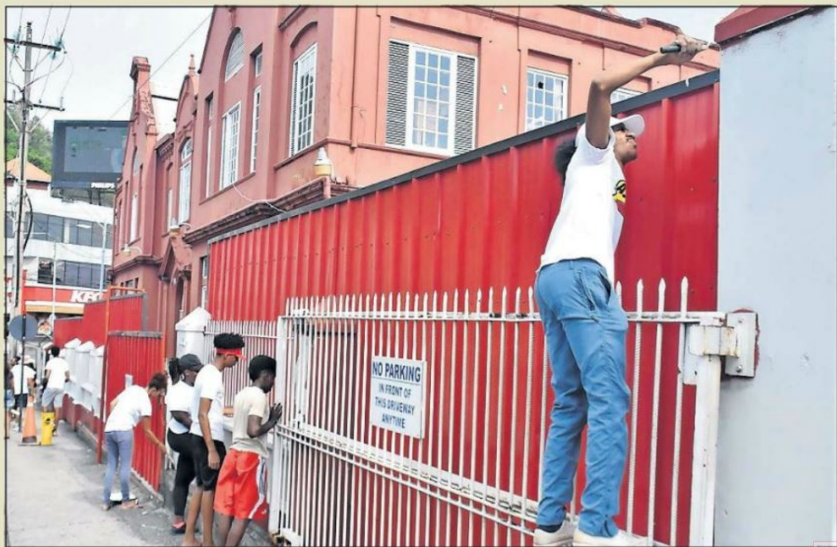
SANDO SPRUCE-UP: Volunteers from The University of the West Indies (UWI) paint the perimeter wall of the Carnegie Free Library at Library Corner, San Fernando, on Sunday. This was part of the effort by the San Fernando City Corporation to enhance the appearance of the city centre. —Photo: TREVOR WATSON
