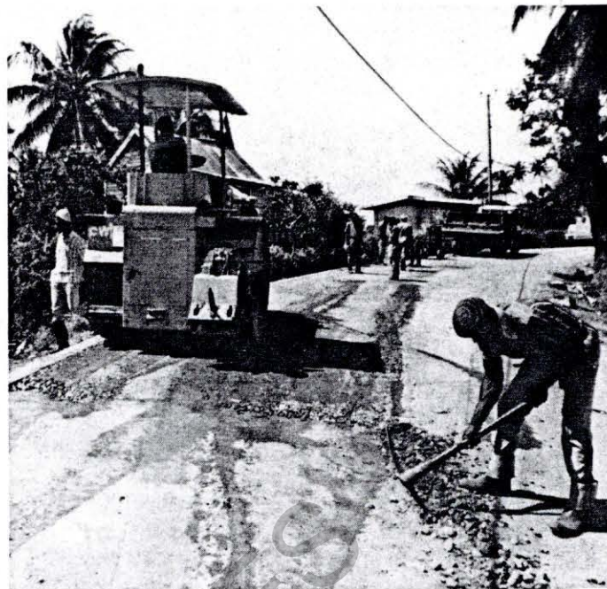
Surfacing a section of the EDF-financed Eastern Main Road
