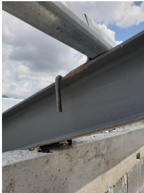
Figure 52: Conn. type 2b on a house in Barataria, Trinidad
