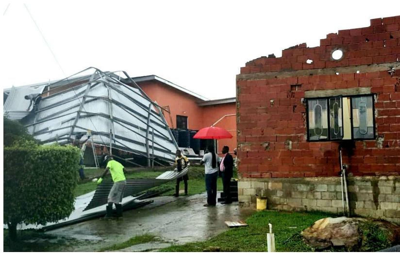
Photo 1: Entire roof blown off in Point Fortin Trinidad
