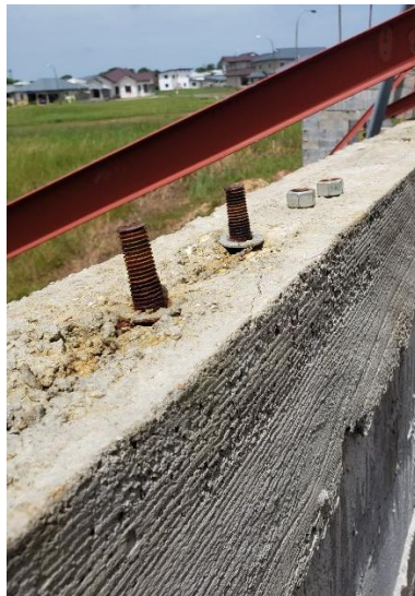
Photo 5: Anchor bolts for Conn. type 1 on a house in Arima, Trinidad
