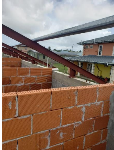
Photo 4: Conn. type 1 on a house in Arima, Trinidad
