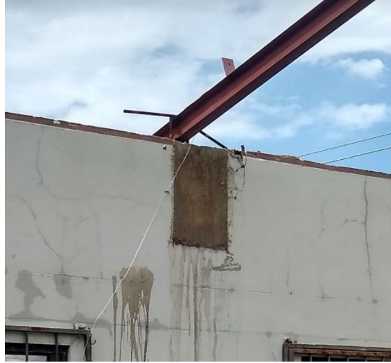
Figure 47: Conn. type 2 on a house in Arima, Trinidad
