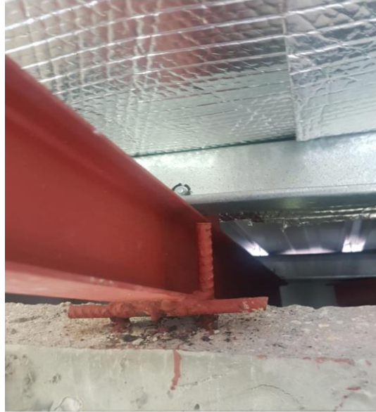
Figure 56: Connection type 3 on a house in Arima, Trinidad
