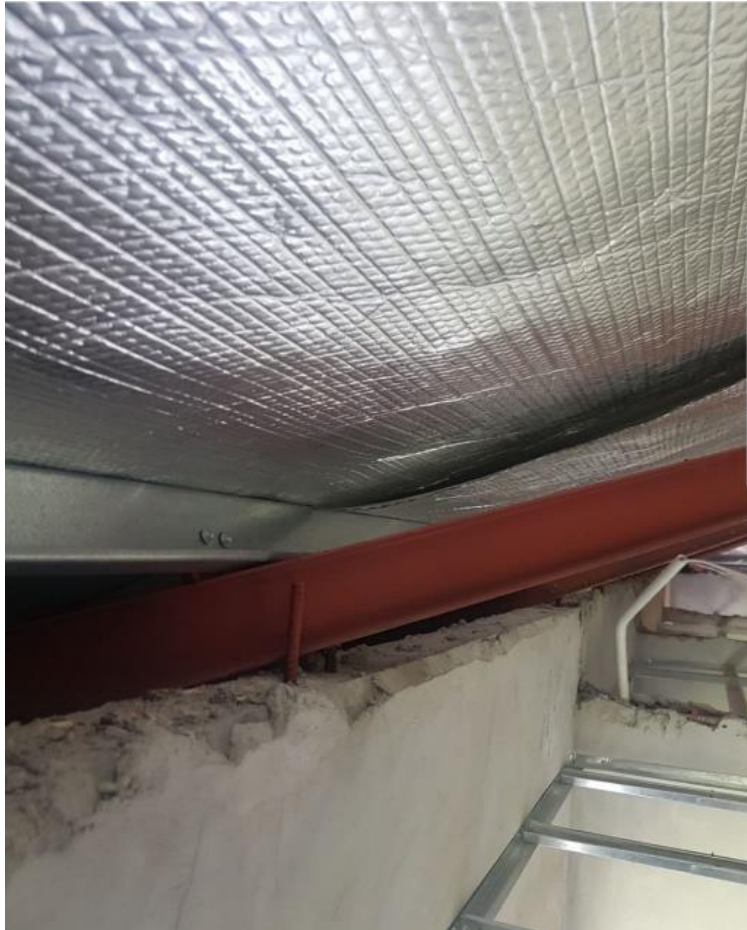
Figure 61: Connection type 3a2 on a house in Arima, Trinidad
