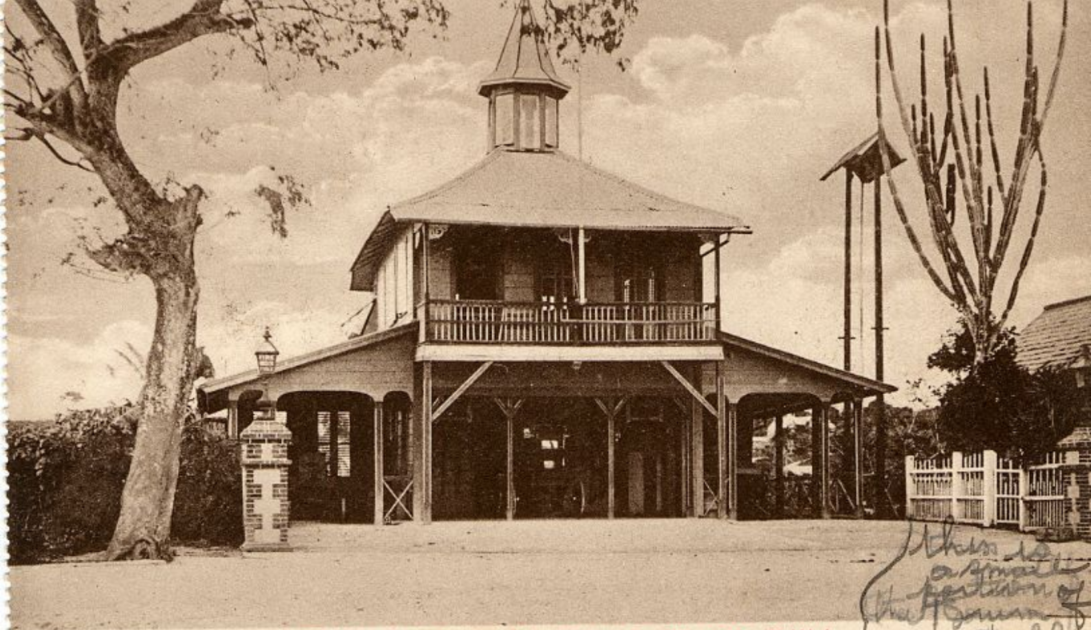
FIRE BRIGADE STATION, SAN FERNANDO, TRINIDAD, B. W. I.
