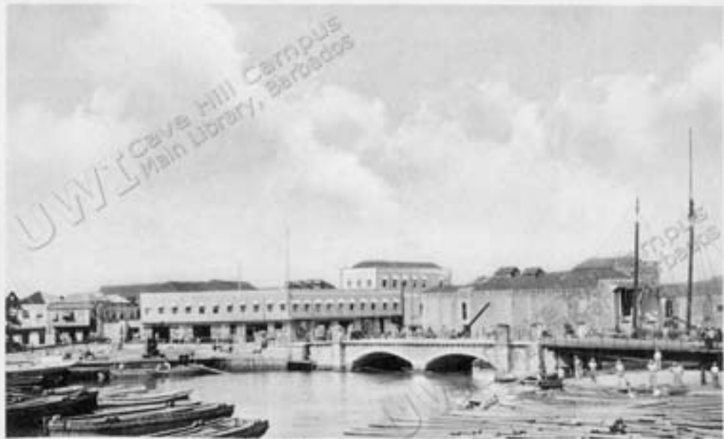
HL4. THE CHAMBERLAIN BRIDGE, BARBADOS.
