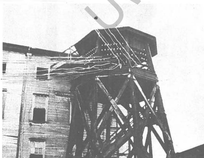
The old Telephone Exchange Cupola, at McInroy's Building, feeding all the overhead lines into city's telephone system. Under the new system all lines will go underground.
