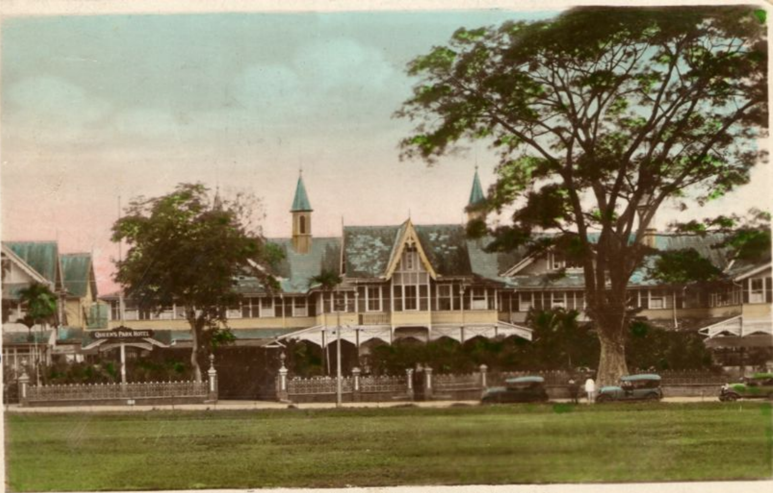
Queens Park Hotel. Port of Spain. Trinidad
