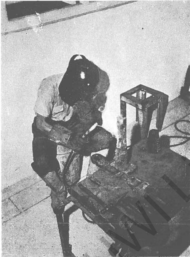
Second Year Apprentice A. Legall Arc Welding.
