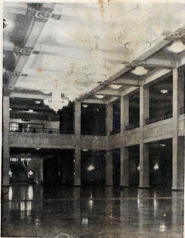
Inside the central hall
