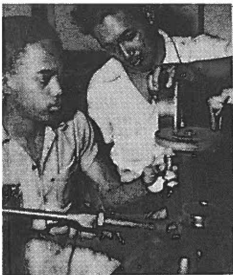
Apprentice Alvin Dorset receiving instruction in Pressure Gauge Calibration from Mr. F. Sucre, one of the Instrument Shop fitters.
