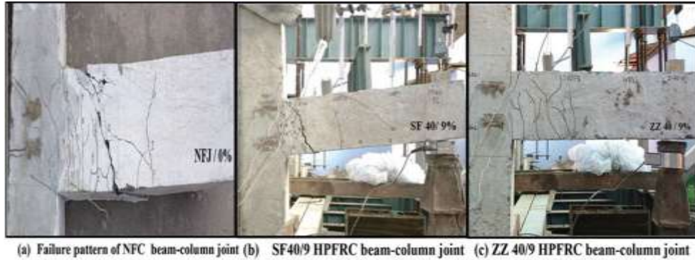
Figure 9: Failure pattern in beam-column joints
