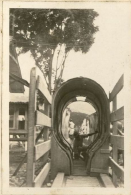
The Spraying Machine showing "entrance" and "exit" races
