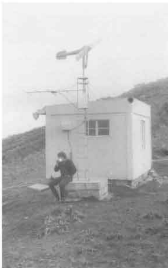
Figure 7: Photograph of the observatory constructed on the crater rim of the Soufrière volcano following the 1971-72 eruption. The photograph shows the wind-dirven electric generator that provided power to recharge the batteries. The building was damaged by vandals and destroyed completely in the early stages of the 1979 eruption.
