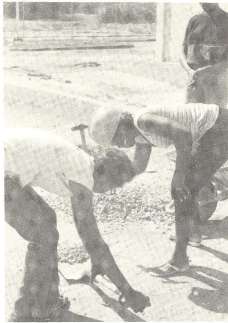
— Preparing to mix cement.
