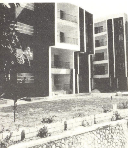
— WCC members helped to construct this apartment block on Old Hope Road.
