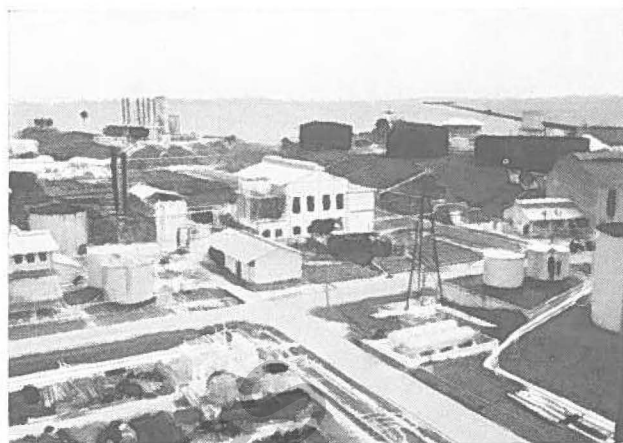
A view of part of the Refinery area taken from Topping Plant No. 3.
