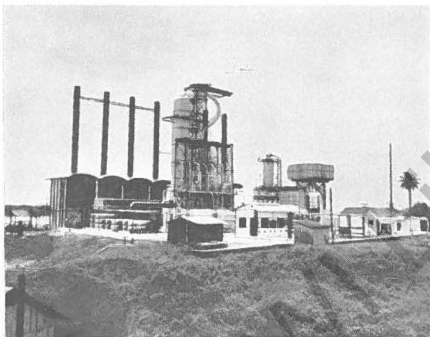
Topping Plant No. 2.
