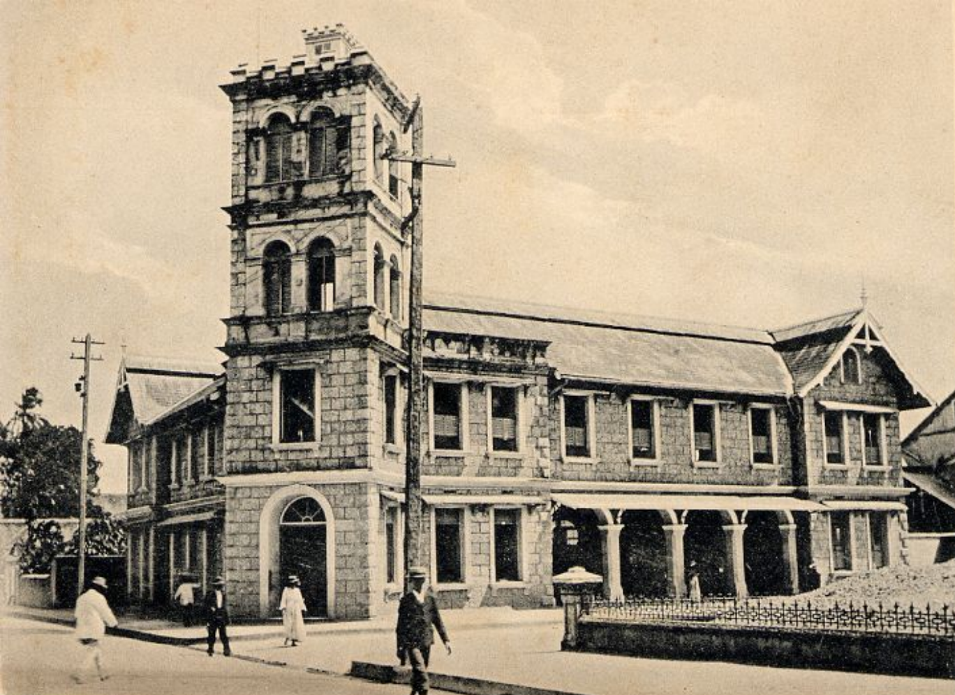
Fire Brigade Station, Trinidad.
