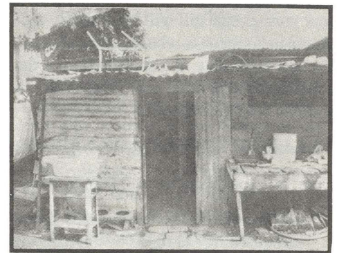
The first property purchased by the co-op awaits renovation (top). Typical shelter conditions for many of the co-op members (above).
