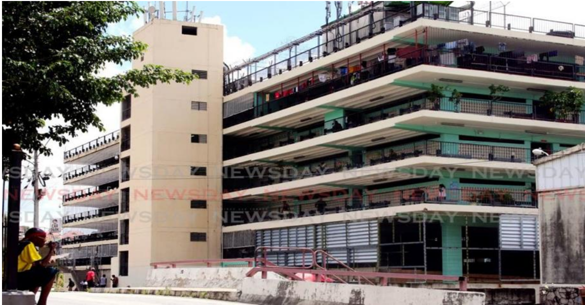
Fig. 1. Riverside Plaza Car Park, Port of Spain, where the homeless are sheltered by the society of saint Vincent de Paul (Cholai).
