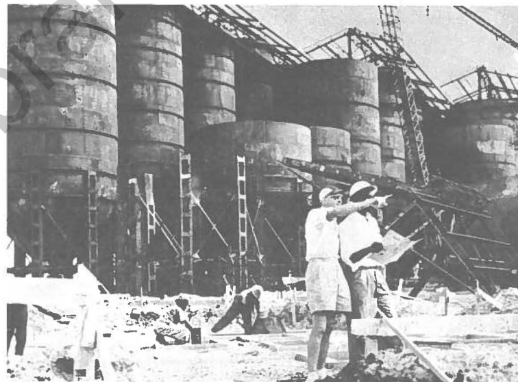
Canadian-born construction Engineer Gerry Gale, in charge of construction works, directing operations with local workmen. In the background are huge precipitators into which bauxite and solution of caustic soda will be poured, to extract the white powder Alumina.
