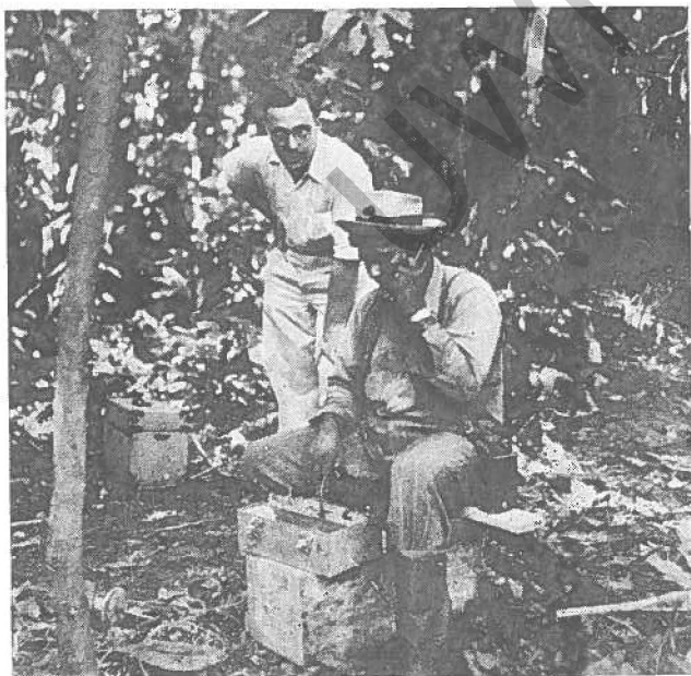
Here we see the shooter waiting for the final order to explode the dynamite by means of the shooting box in front of him.
