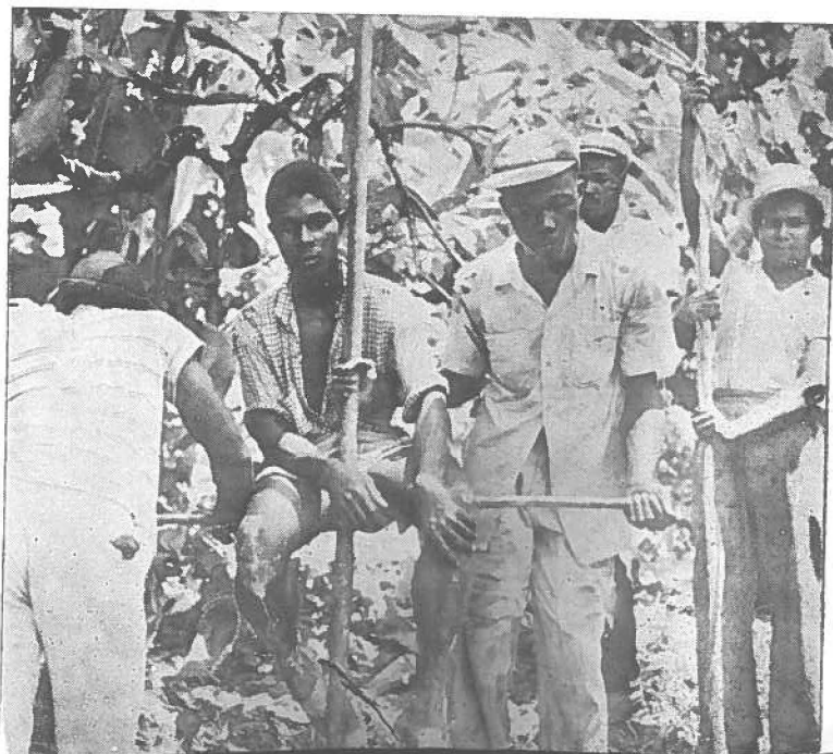
Another view of drilling operations showing drill stem being rotated by hand. Note man sitting on chain tongs to give weight.
