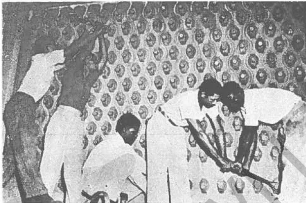
This is not the Boscoe Holder Troupe of dancers but a group of Refinery Boilersmiths tightening handhole caps on one of the water tube boilers.
