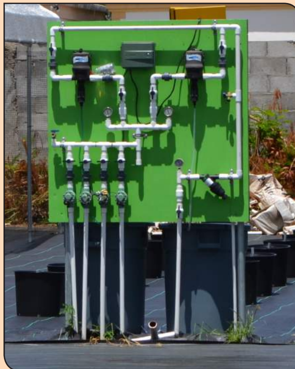
Figure 10.6B: Outdoor irrigation controller
