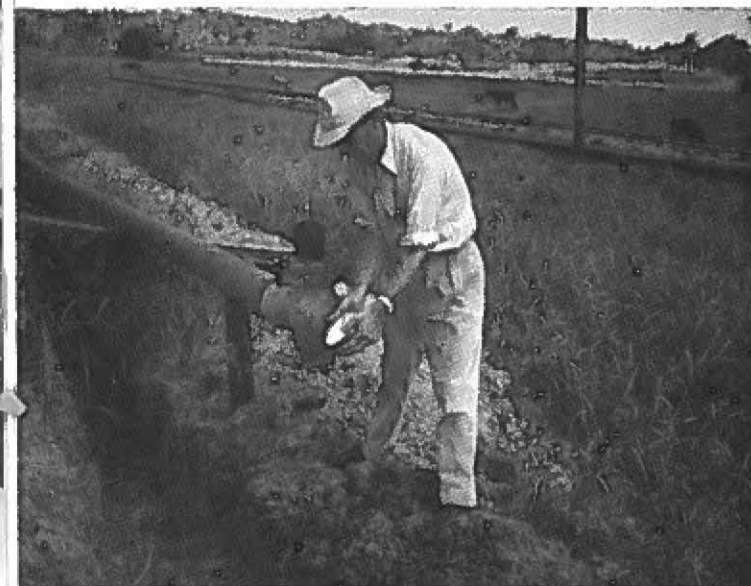
Below, Mr. M. Zaneta places a gauge on a section of the line before carrying out a water pressure test.
