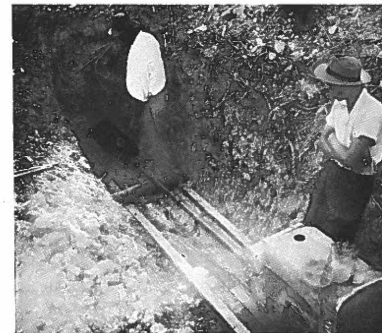
An earth auger (above), made in our workshops, tunnels under a railway embankment boring a hole through which the line was subsequently passed. Below, an angle-bladed tractor back fills the ditch in which the pipe has been laid.
