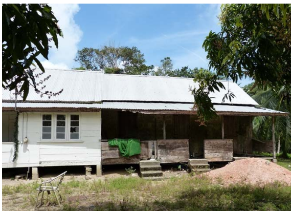
(Fig. 18) Barracks , Mahabir
