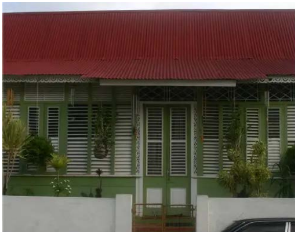
(Fig. 6) House with Jalousie Windows and Doors , Waldron
