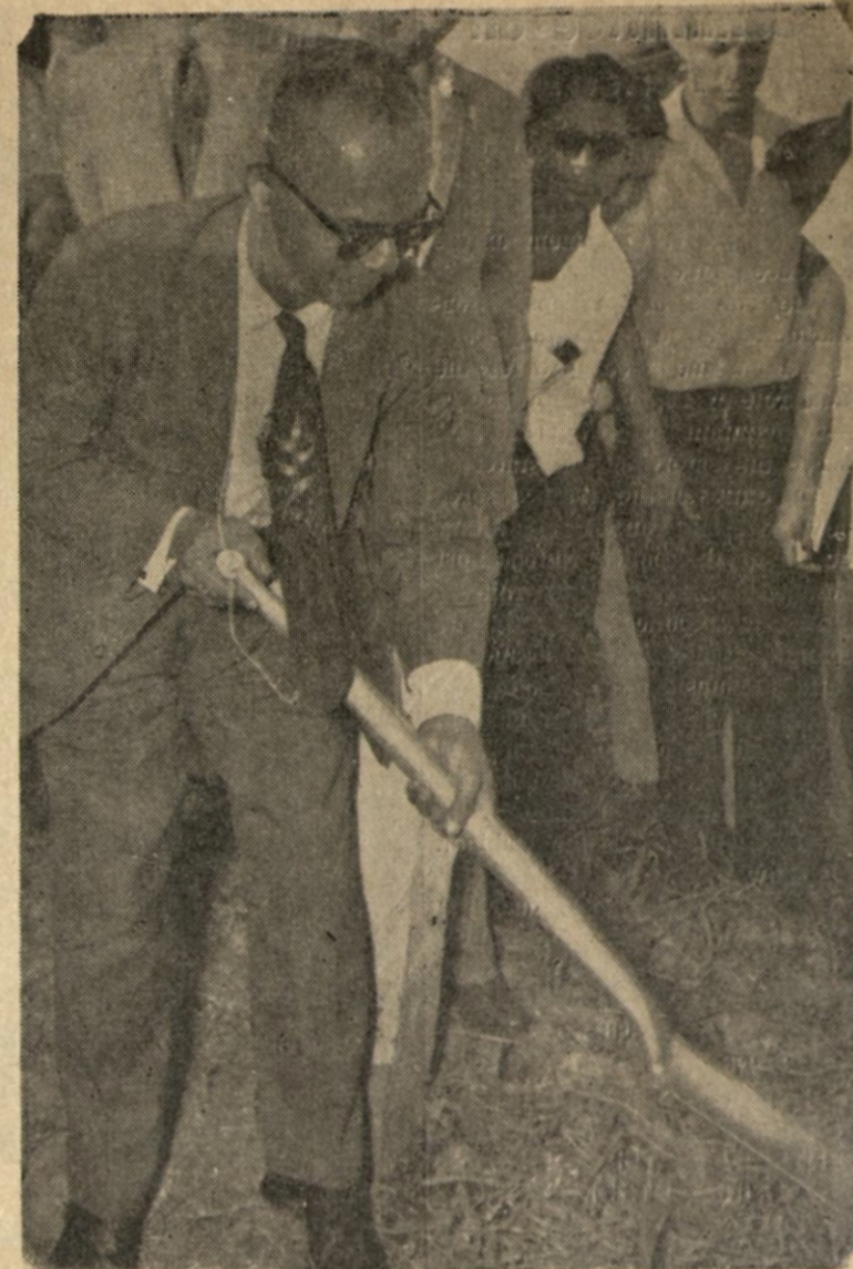
The Prime Minister, Dr. Williams turning the first sod on December 22, 1961, to launch the $2m Oropouche Reclamation Scheme.
