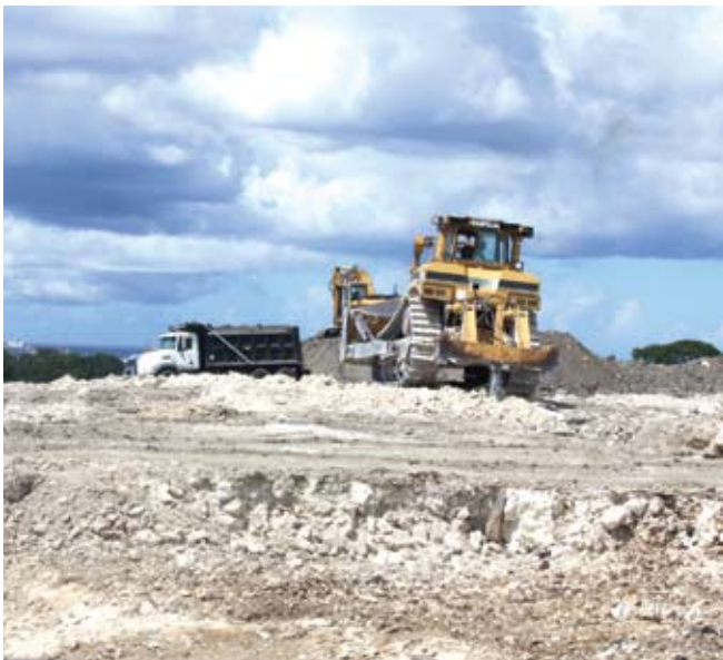
Earth moving works started on CXC 's new Headquarters site in mid October
