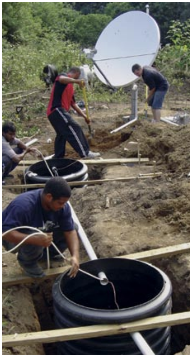
Technicians install VSAT equipment as part of a project to upgrade the seismic monitoring network.
