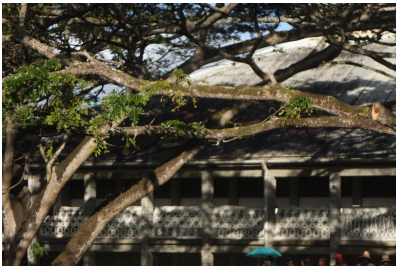
Figure 24 Covering of Open Campus Railings, Xavier Kistow - Davis 2023
