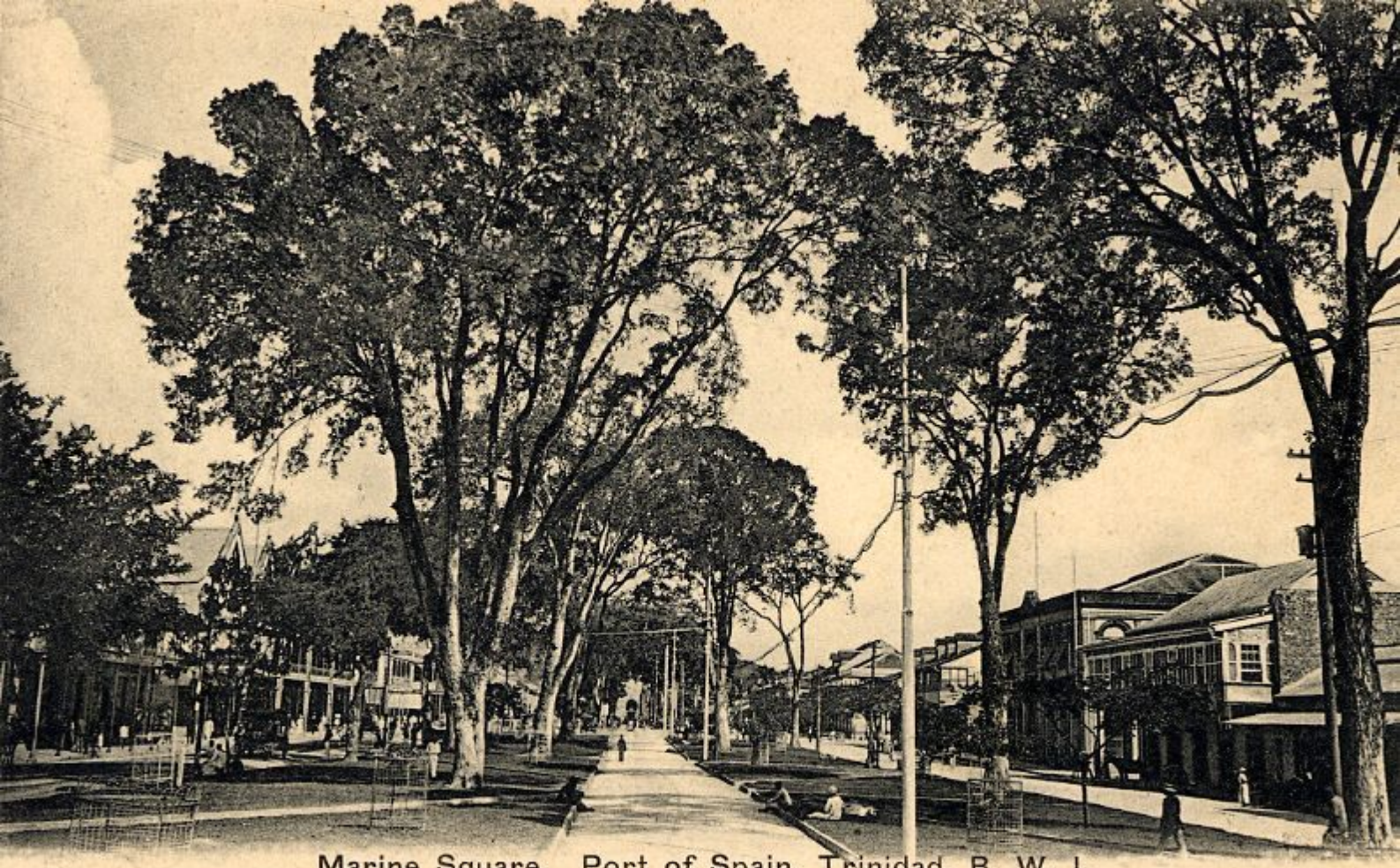
Marine Square. Port of Spain. Trinidad, B. W. I.
