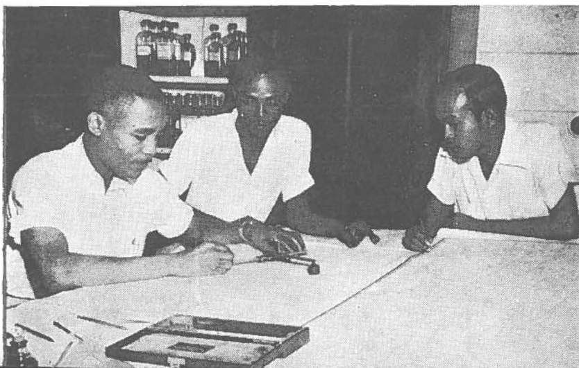
The Section Head of the Topographical Section, Mr. S. E. Morris, calculating an area with the help of the planimeter. The two draughtsmen looking on are Mr. W. L. B. Furlonge (centre) and Mr. H. Rampaul (right)
