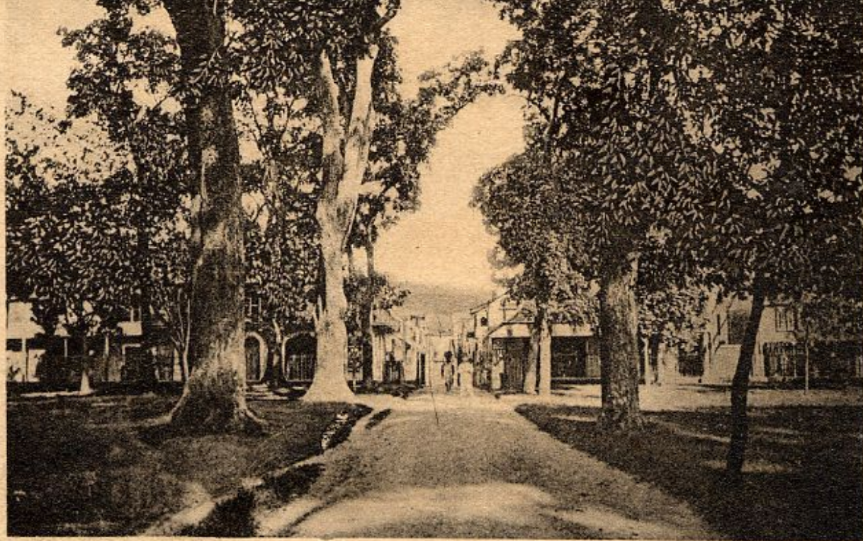
Port of Spain, Trinidad. Brunswick Square.
