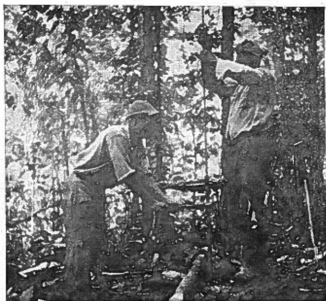
Drilling auger holes for test purposes.
