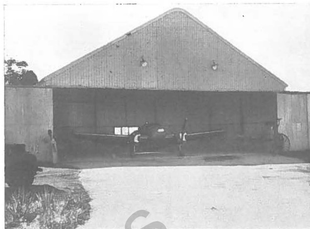
The Hangar at Point Fortin.
