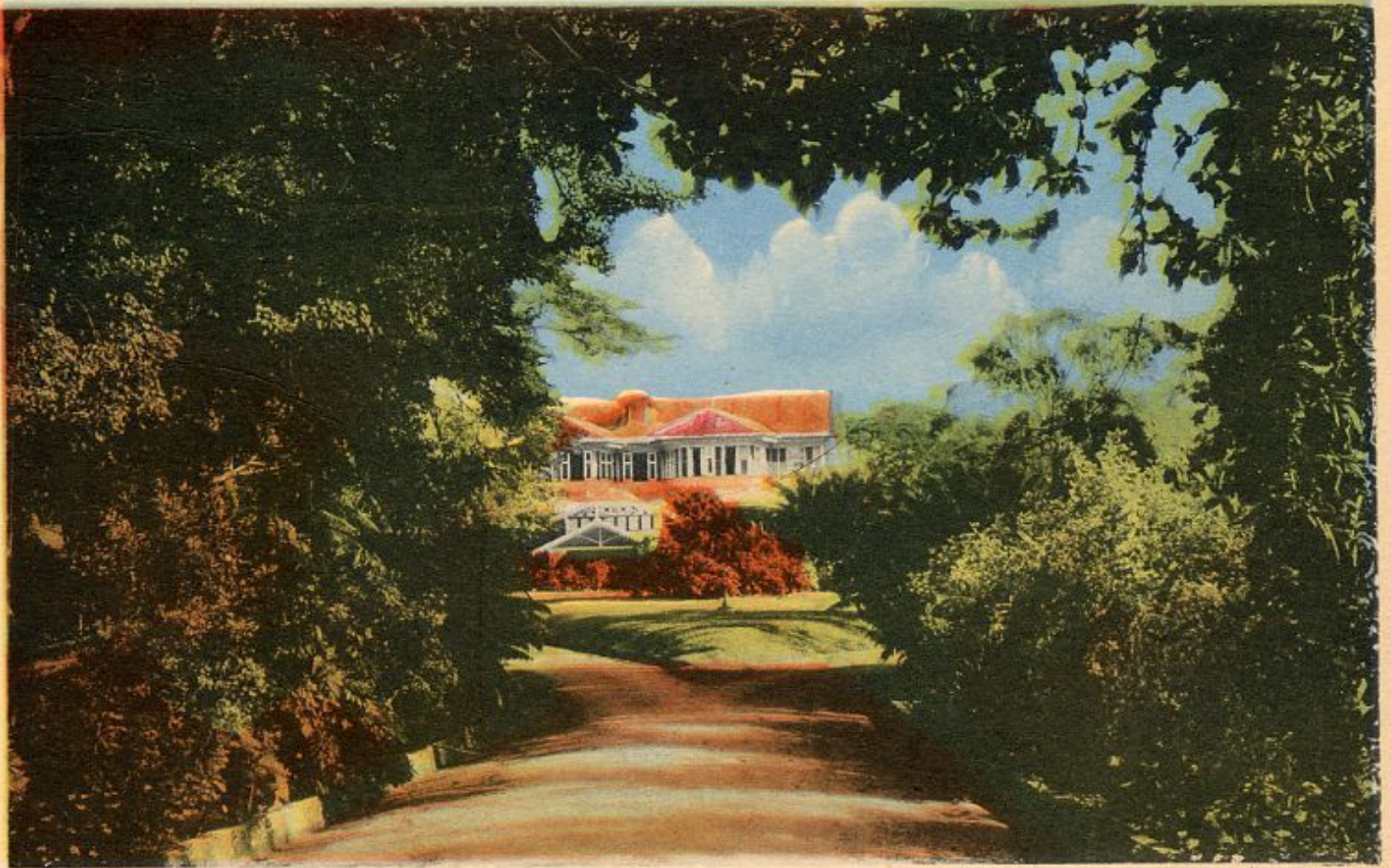
Private Residence, Port-of-Spain, Trinidad, B.W.I.—20793.
