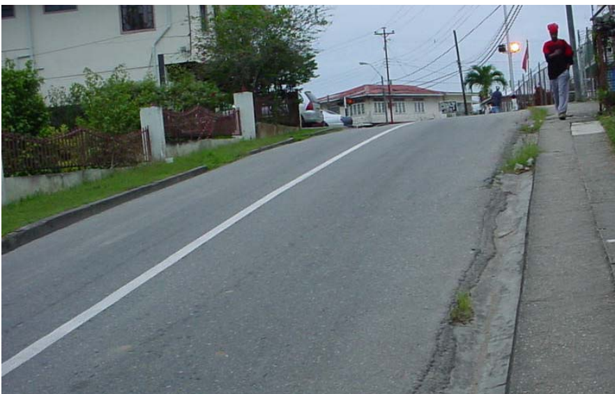
Figure 2.5: Crossing obscured by adverse vertical alignment (sharp vertical curve)
