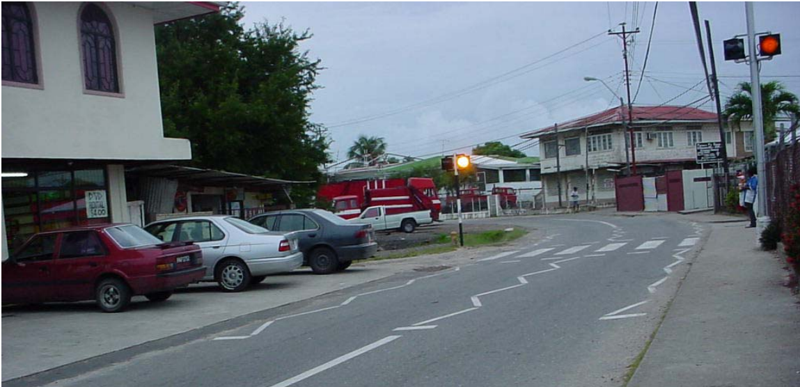
Figure 2.4: Crossing obscured by adverse horizontal alignment (sharp horizontal curve)
