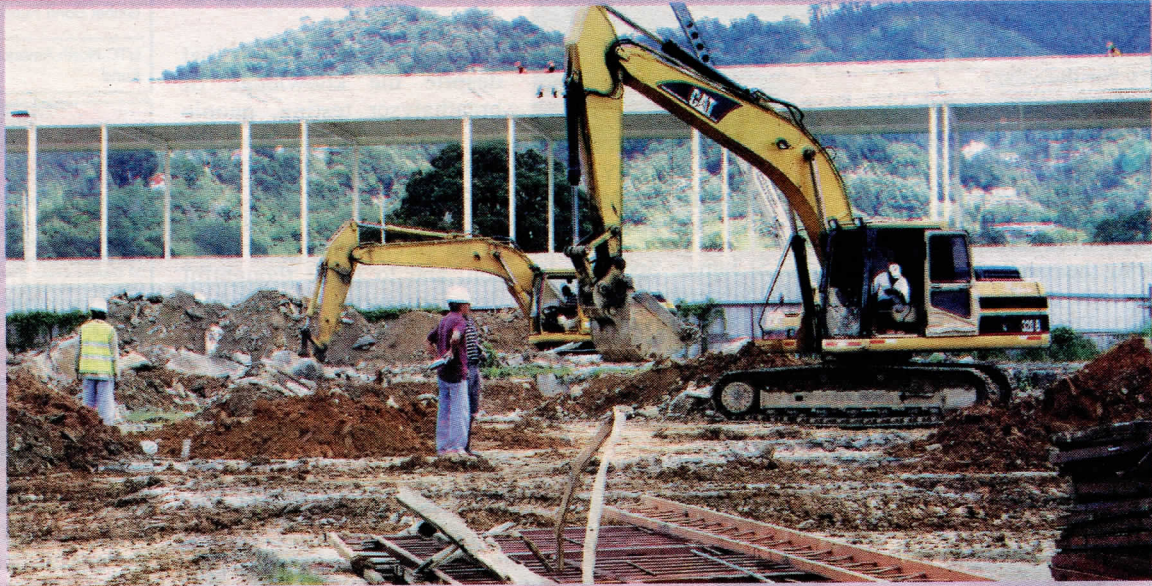
HEAVY MACHINERY: Work at the Queens Park Savannah well on the way for Carnival 2011. In the background is the new North Stand and the foreground where the stands will go up. PHOTO BY SUREASH CHOLAI
