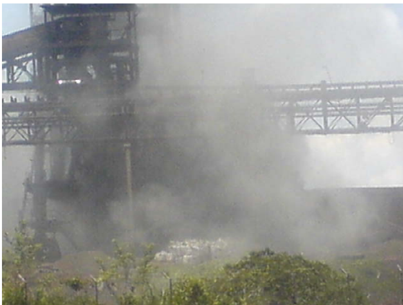
Fig. 8 Typical visible emissions from Direct Reduced Iron (DRI) plant of NuIron Corp. in Trinidad/Tobago, 2008. Photo by Ryan Sant.
